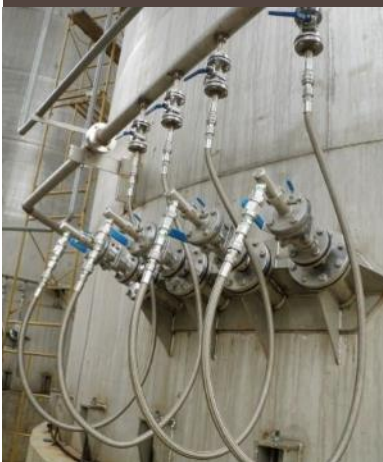
HyperSpargers™ oxygen addition
